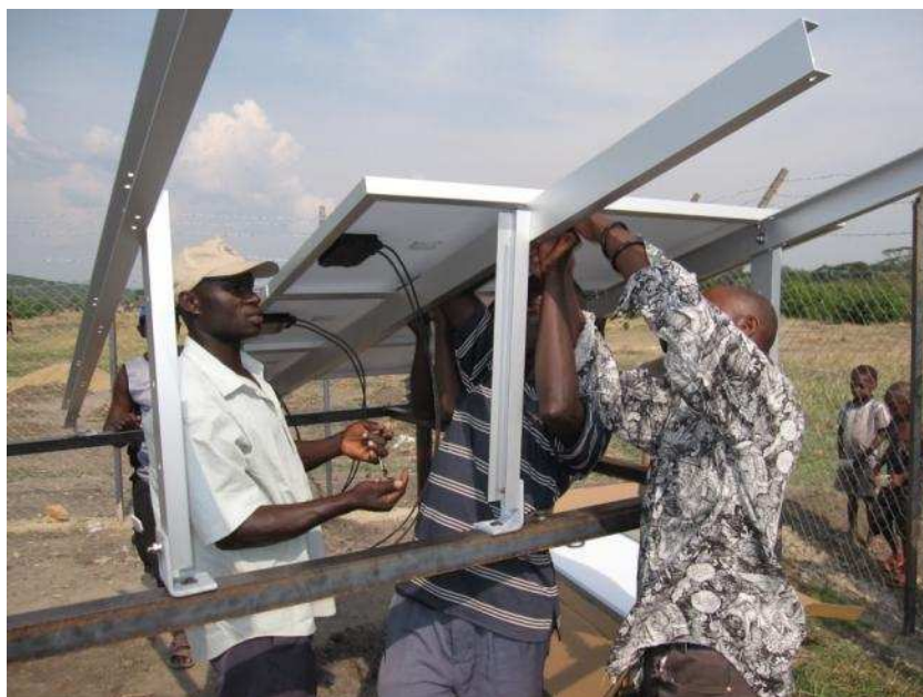
Installation of solar panels
