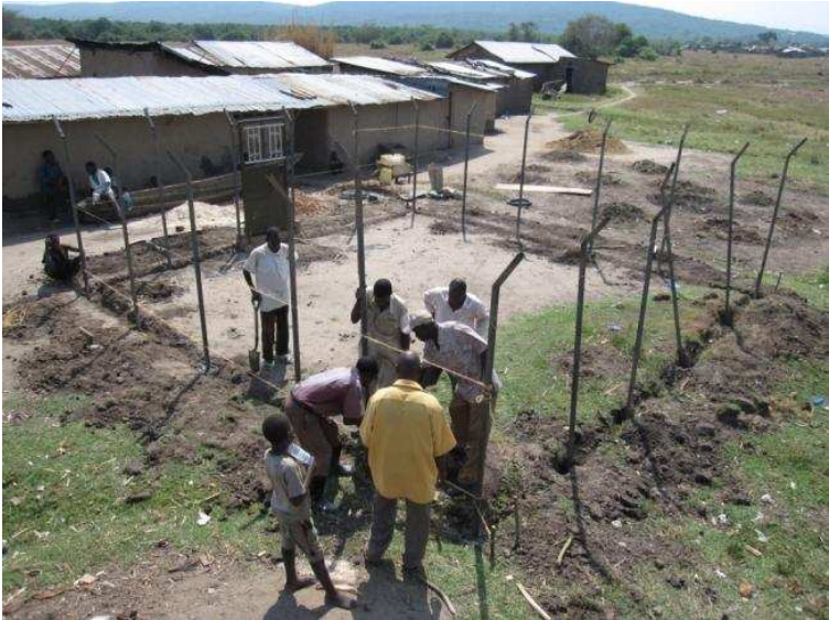
The fenced compound for the solar panels being constructed.
